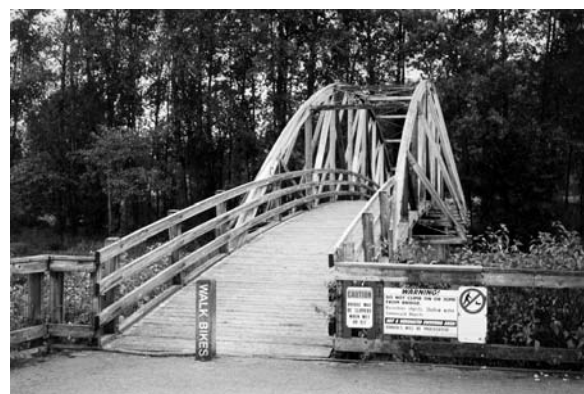
Pedestrian Bridge Over Sammamish River
