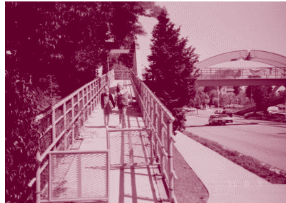
Ramp Leading to Overhead Crossing in
