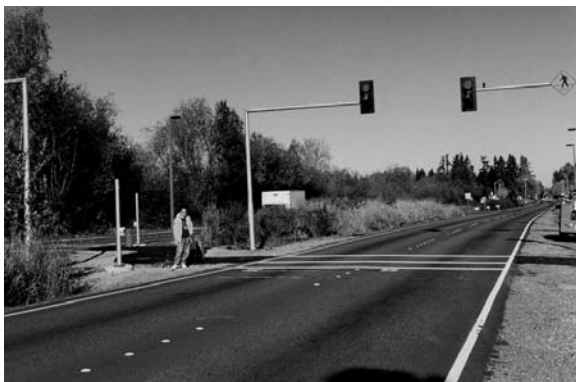
Pedestrian actuated signals at mid-block crossings only operate in the presence of foot traffic. Notice how median path directs pedestrians to look at oncoming traffic.
