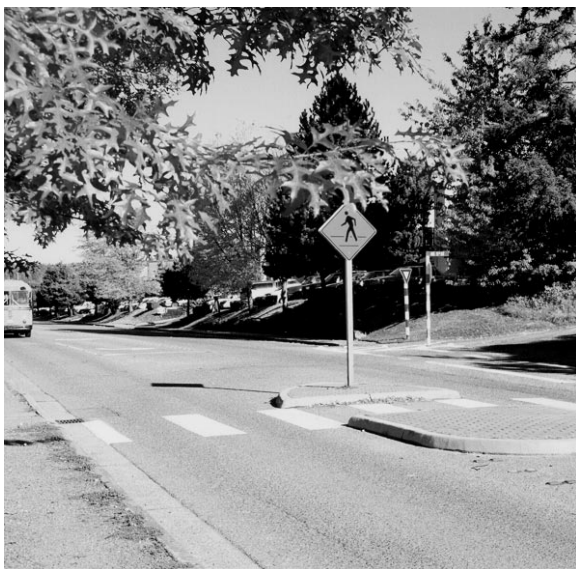
Mid-block crossing with median refuge island.
