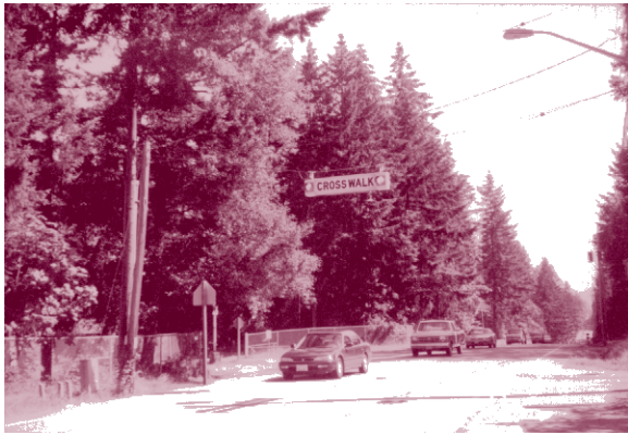
Overhead Flashing Beacon
