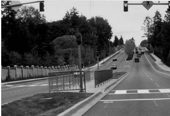
Railing is used to channelize pedestrians so they can view oncoming traffic.
